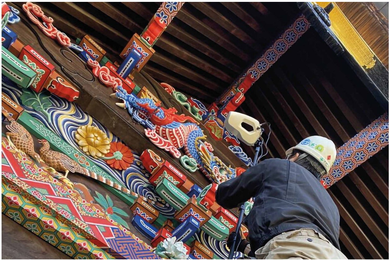
Cover: Full-color 3D printed replica of "Tsunagi no Ryu" modeled on the 3DUJ-553
